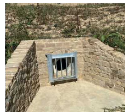
Stone clad headwalls.
