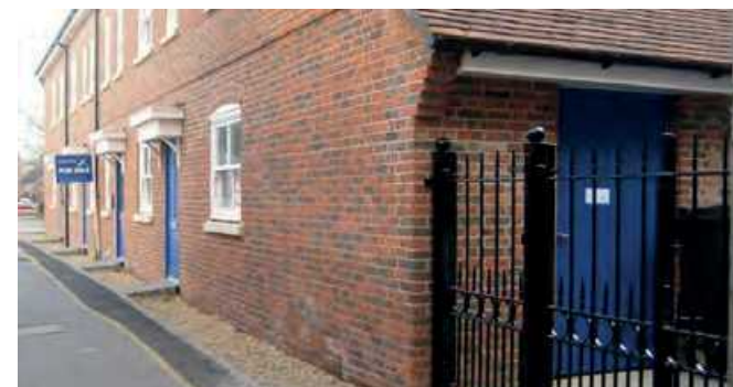
Communal bin store integrated into a lean to behind a security gate. A visible side wall on a corner plot is finished in local stone to a high standard.
