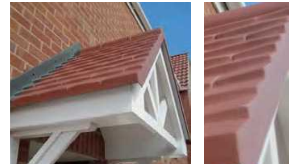
Above: Mass produced materials like moulded glass reinforced plastic (GRP) are inauthentic, appear crude and undermine the quality of the development.
