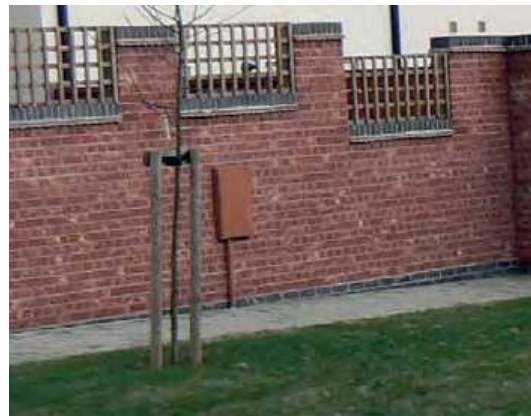
A meter box positioned on a rear boundary wall to an internal parking court and colour coded to the brickwork.
